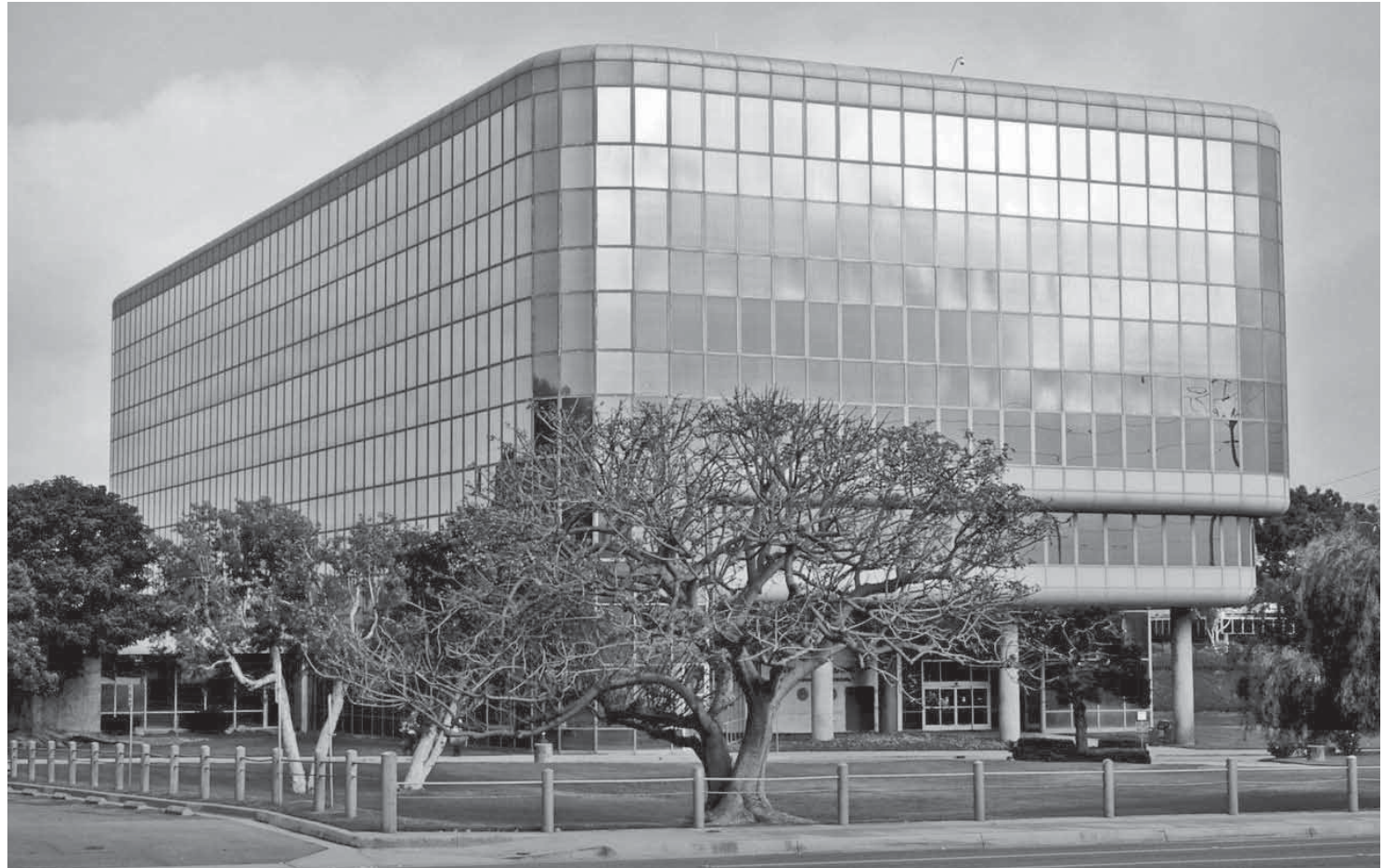
A well known and characteristic landmark in Lawndale, The Federal building at 150000 Aviation Blvd., houses the Federal Aviation Administration's West Coast Headquarters. The building was the first-designed Southern California building to have a mirrored skin. The mirrored glass skin became ubiquitous on corporate architectural designs of the 1970s and 1980s. Photo by www.christopherbarnesphotography.com.
